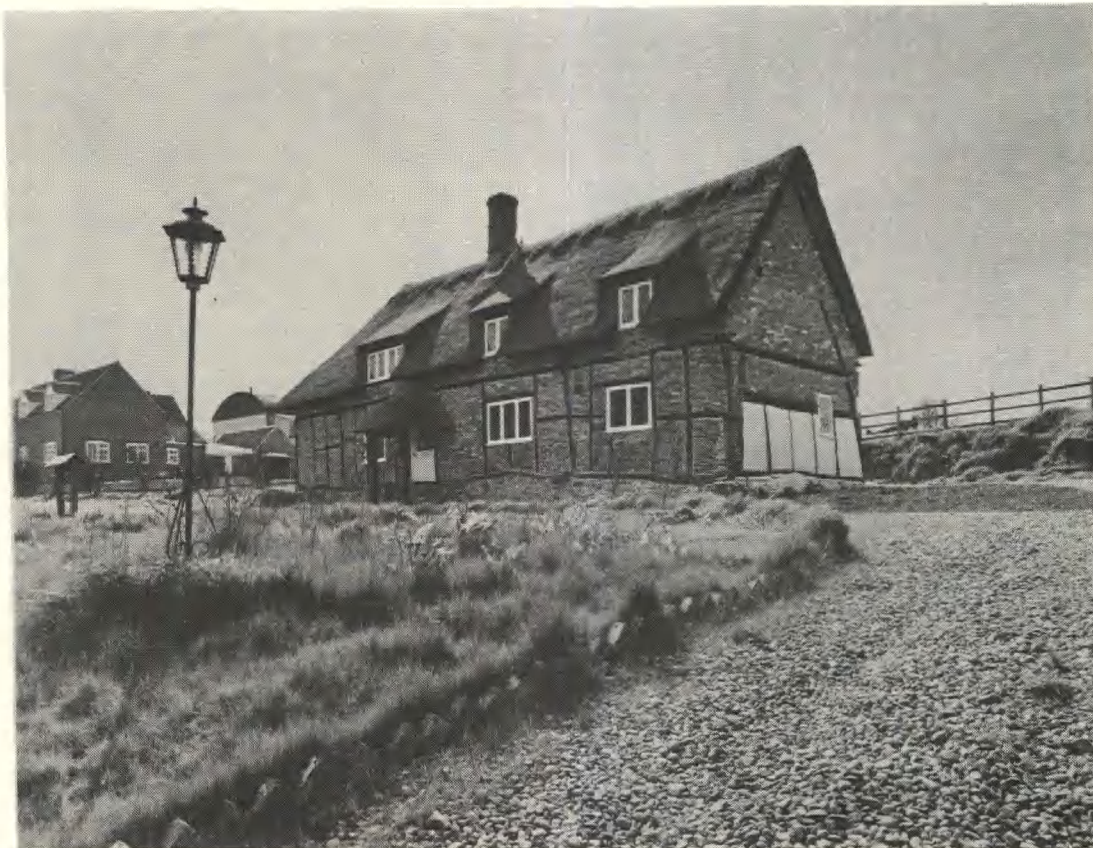
Pl 8 Exterior from north-east after conversion, Husbourne Crawley.
