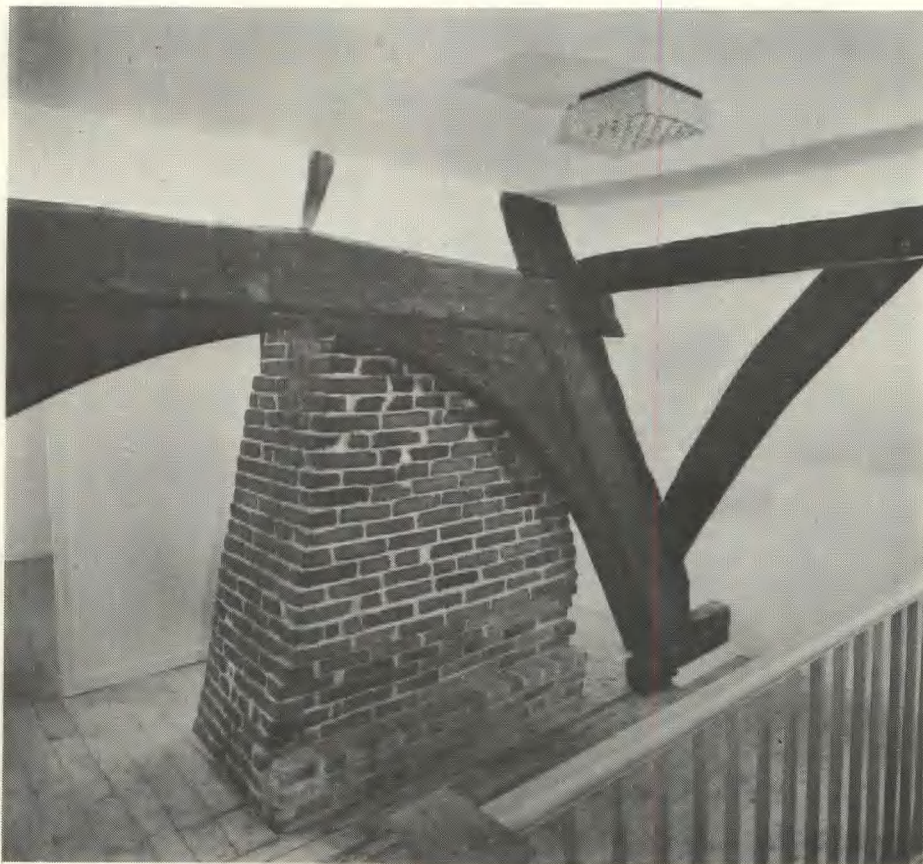
Pl 6 Detail of hall cruck, Husbourne Crawley.
